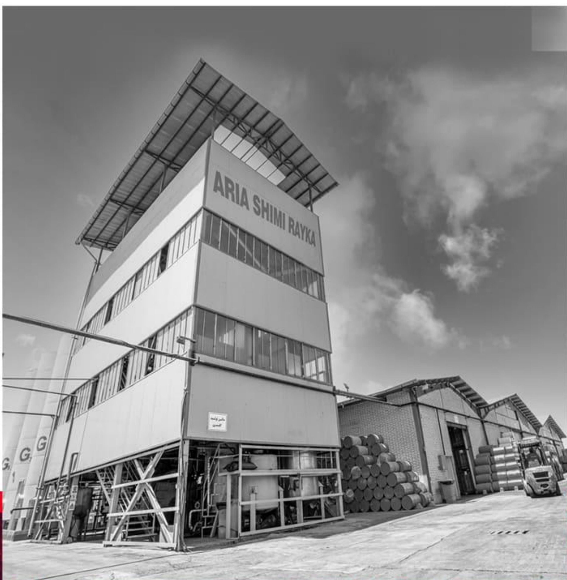
GLYCEROL PRODUCTION PLANT
